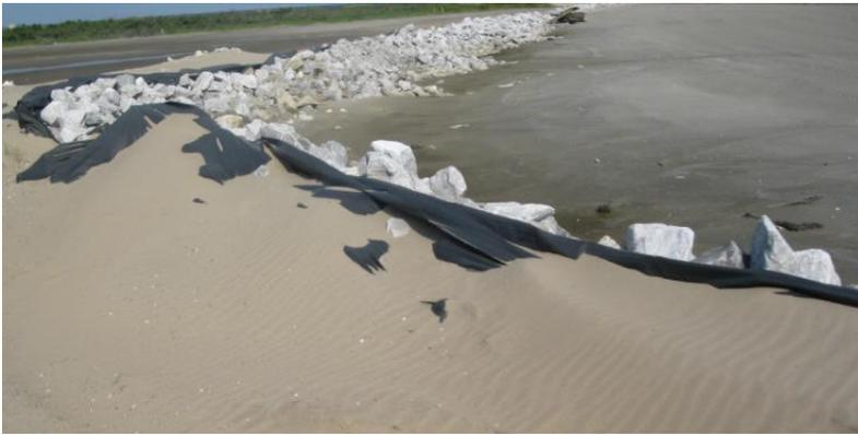
Geotextile barrier held in place by imported rubble across a low section of a barrier beach.
