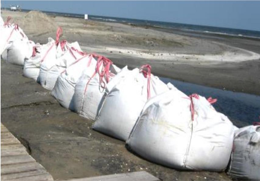
“Super sacks” placed at the high water level across a low point in a barrier beach where waves can wash over into the backshore on spring tides or during storm surges.
