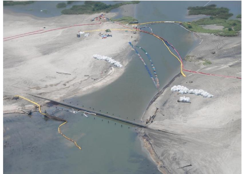
Solid sheet pile barrier under construction across a shallow channel. In the ground view at left, note oil in the lower half of the image. Hard booms, Super Sacks, and snare booms were deployed prior to completion of bulkhead construction.
