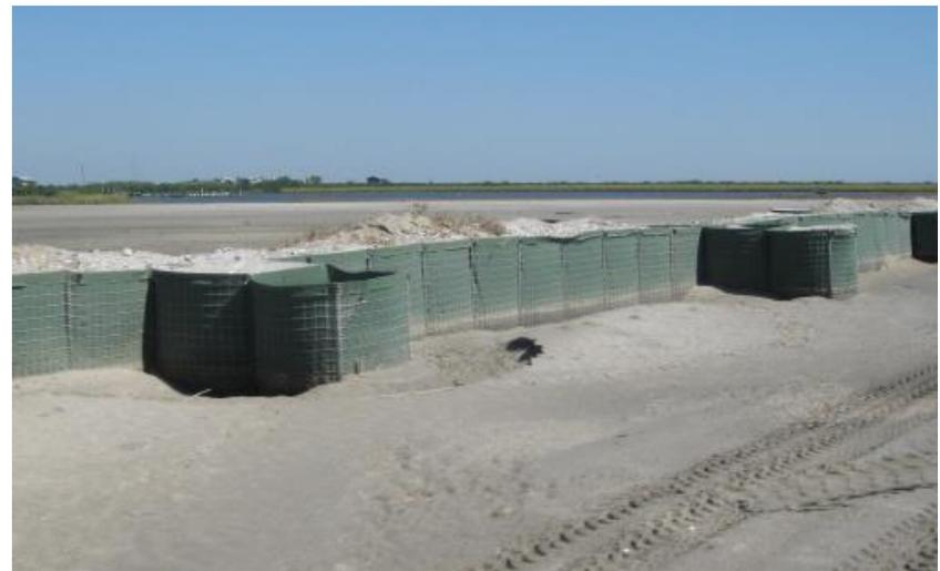
Armored baskets placed along the highest elevation on a long, low sand barrier.
